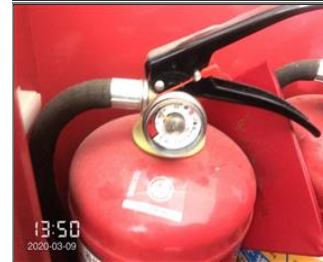
Photo of fire safety equipment Fire extinguishers with proper pressure.JPG
