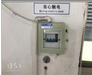
Photo of non-conformity NC Distribution box without cover.JPG
